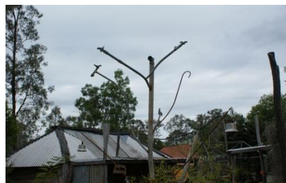
So wet even the water pipes are growing!!
